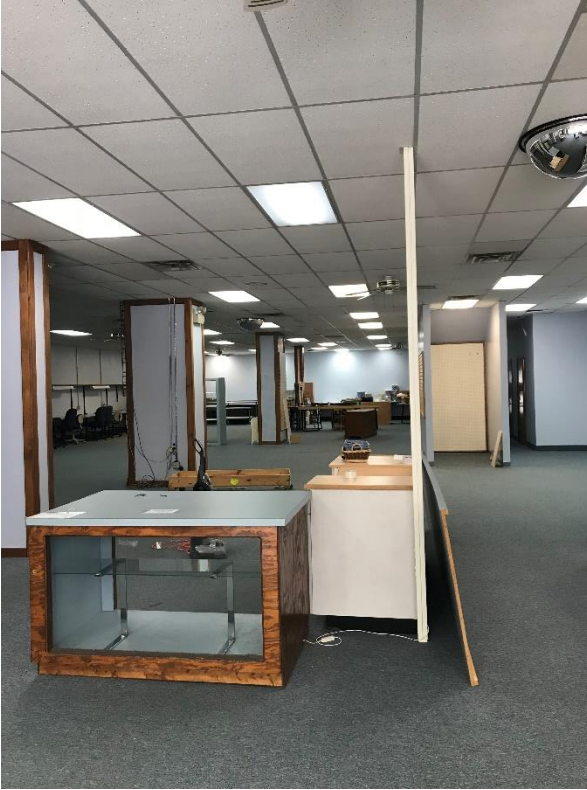
Install POS & refurbish checkout area
