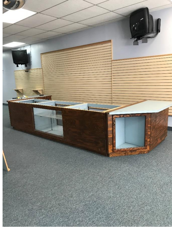
Install wine coolers & refurbish tasting bar area
