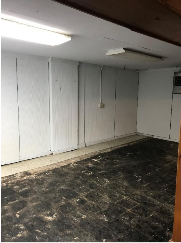
Resurface basement floor to meet ATCP code
