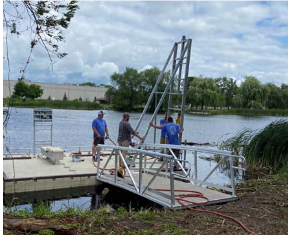
Lakeside Park – ADA Kayak Launch Installation
