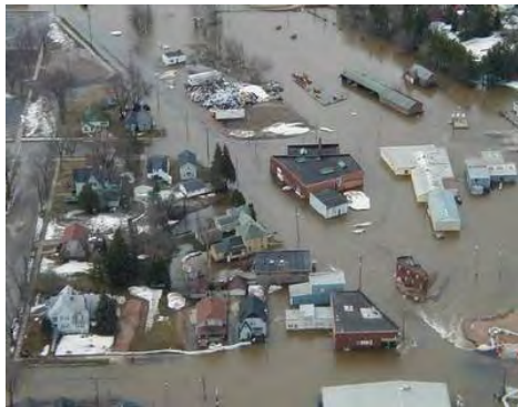
Flooding in Antigo, 2004
