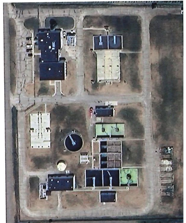
Antigo desires to understand how increased flows and loads from Sartori Cheese could affect liquid and biosolids treatment processes, and the corresponding costs of necessary improvements.
