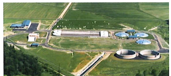
Marshfield Wastewater Treatment Plant.
