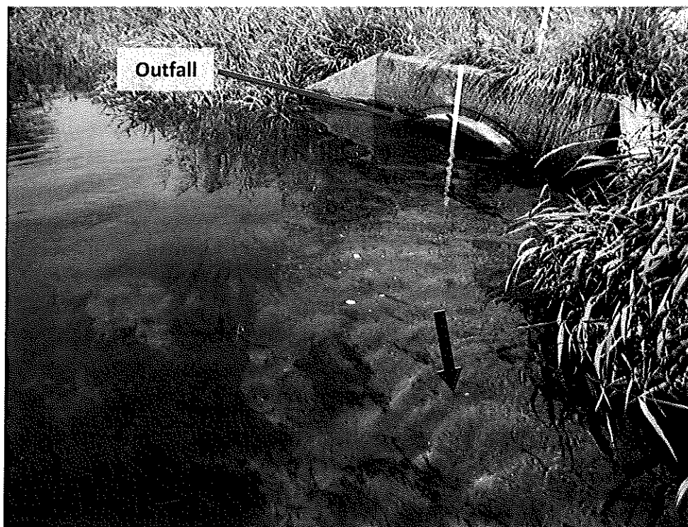
Figure 3: Close-up of Antigo WWTF Effluent Outfall
