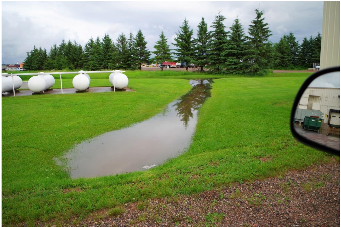
Waukesha Bearing Storage Tanks Looking East
