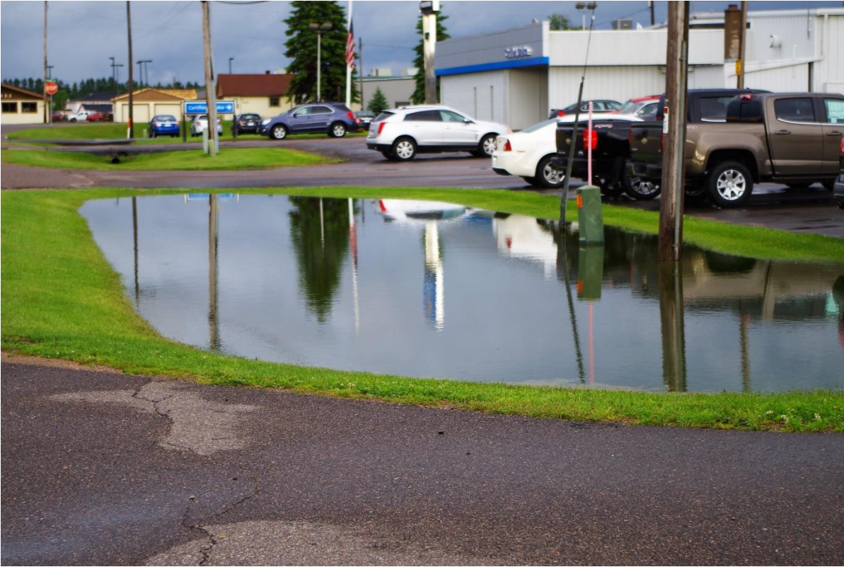
Waukesha Bearing Driveway Looking East
