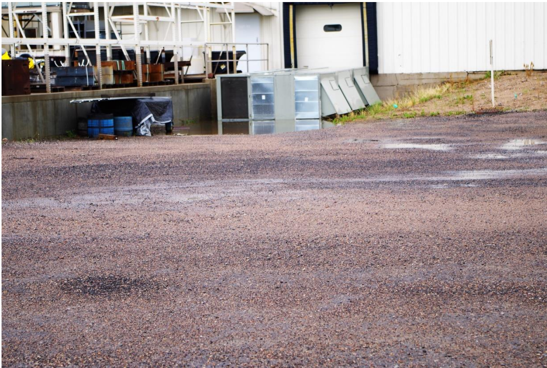
Plaspak Loading Dock Looking North
