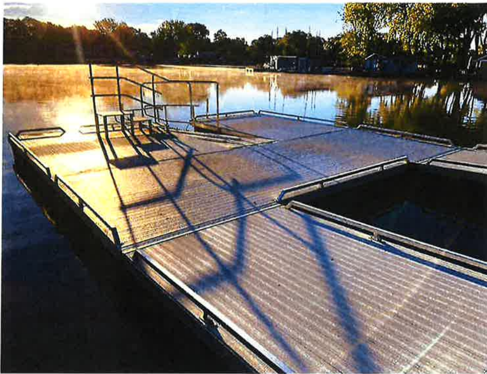
Overall view of ADA canoe and kayak dock/launch.
